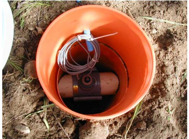
Meter installed in saddle in "bucket" vault.
